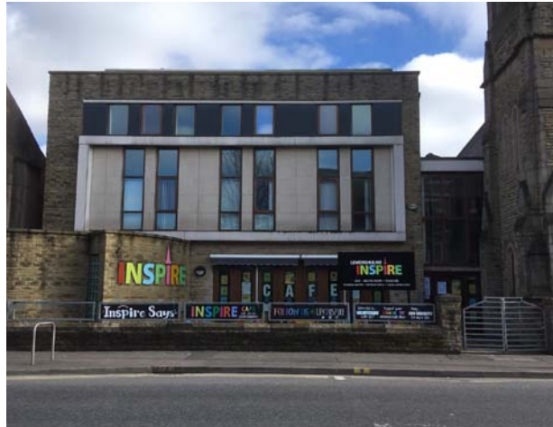
Figure 13: Inspire Centre, with the adjoining church tower on the right.
